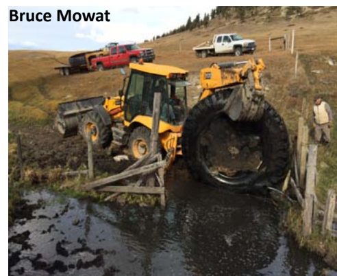
Removing the old trough from the spring.
