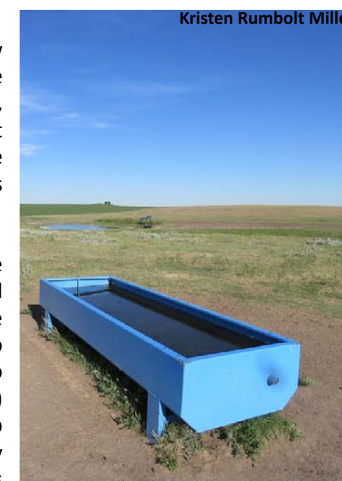
Pipeline from dugout to trough using solar powered pump to trough #1
